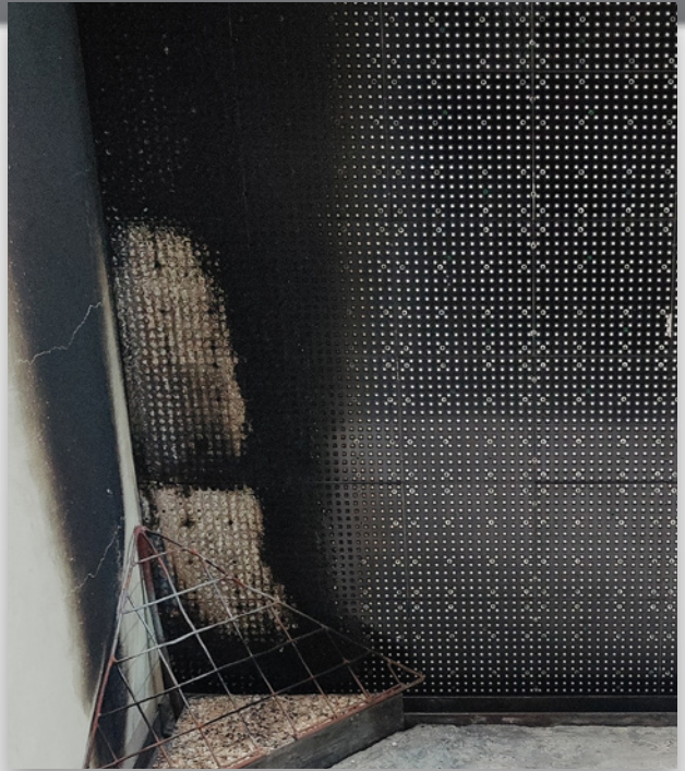
Fig.: SPF equipped LED screen after fire test (SBI)
